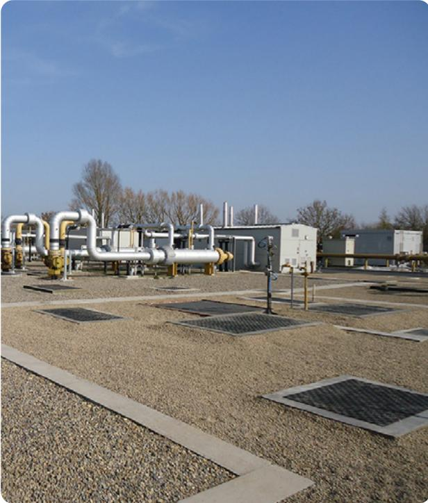
The Fibrelite B125 (12.5 tonne) load rated lightweight trench and access covers
