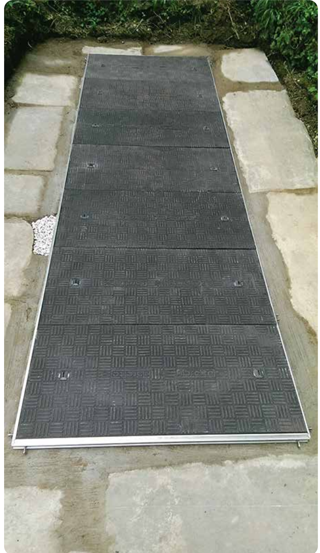
Chemically inert and corrosion resistant covers
