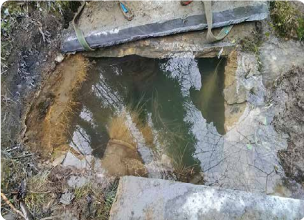
Heavy slate covers were replaced with Fibrelite's lightweight trench covers
