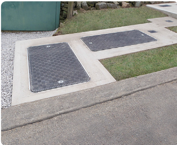
The 25 tonne load tested lightweight covers
