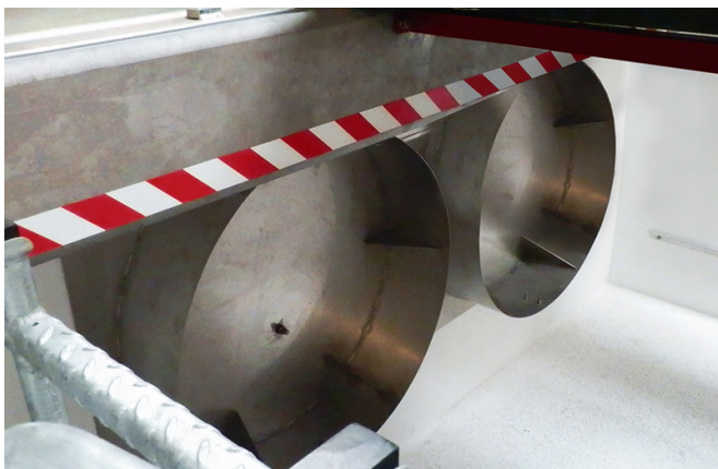
Underground pit to house crane supply lines
