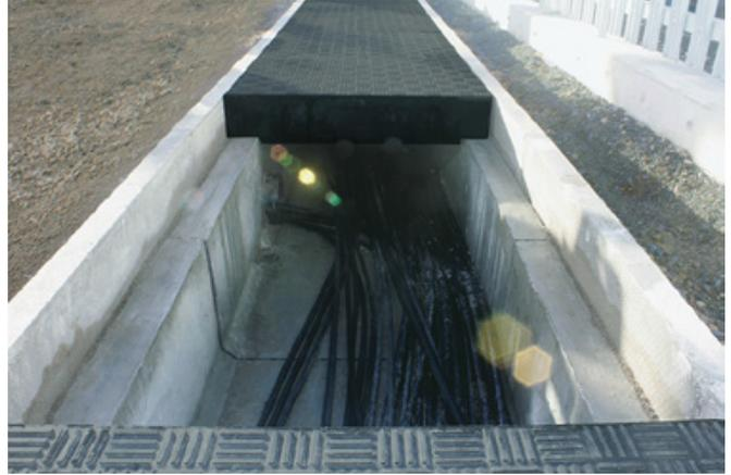
*Slit trench with stepped covers over electrical cabling*
