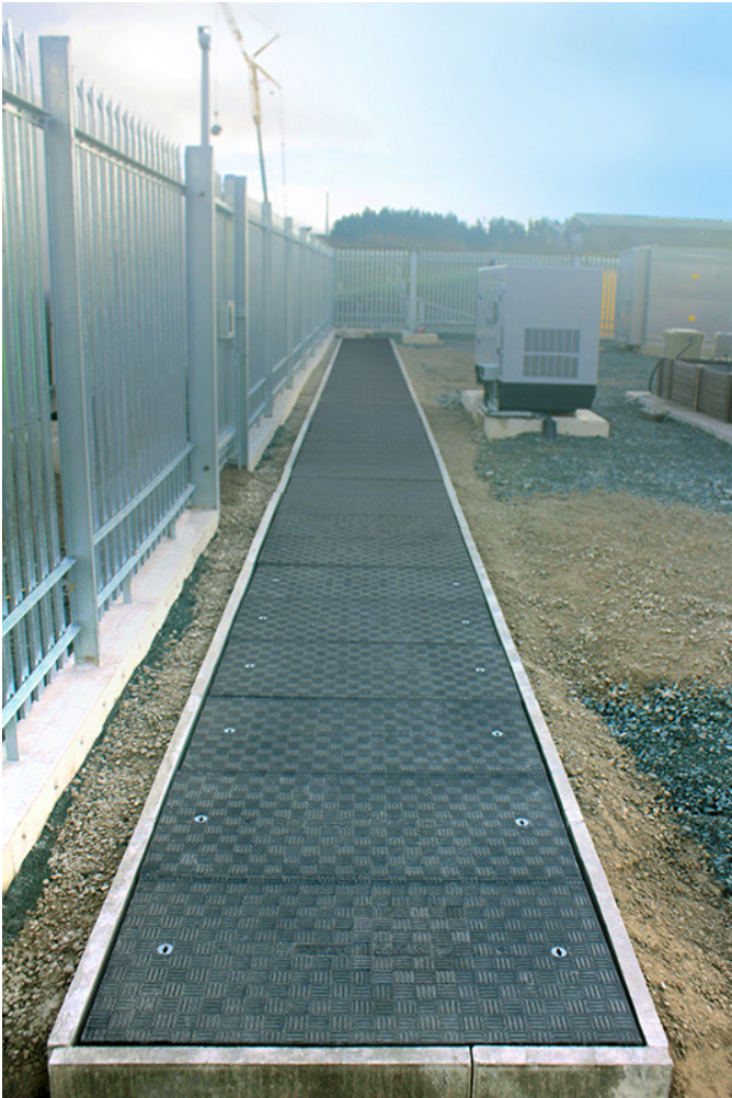
25 metre long pre-cast concrete trench with 1250mm span
