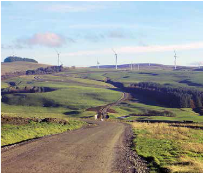
Garreg Lwyd wind farm under construction
