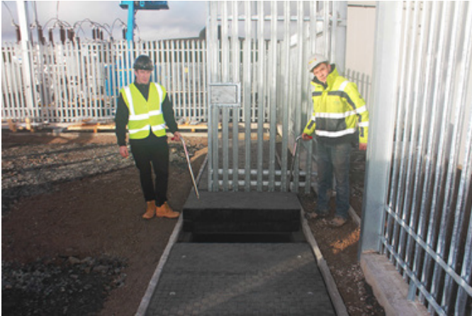
Covers safely manually removed with Fibrelite's ergonomically designed lifting handles
