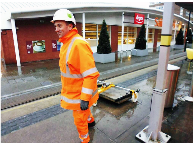
The previously installed heavy concrete covers
