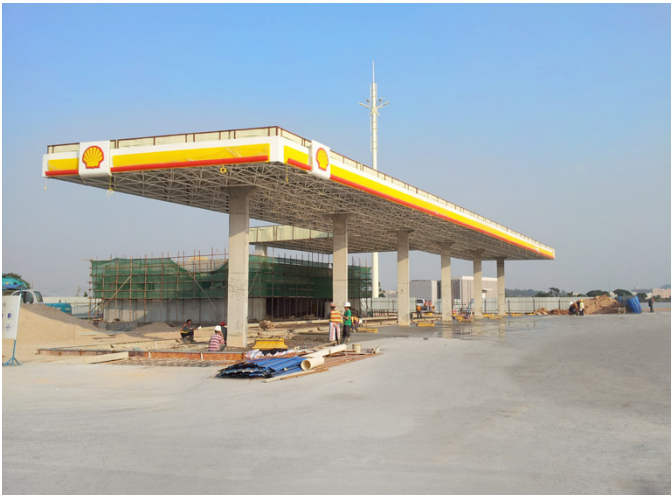
Site under construction
