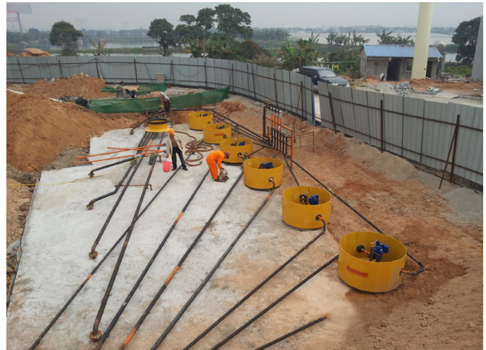
Fibrelite tank sumps (S14-390) being installed
