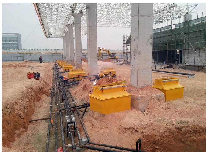
Fibrelite's Gilbarco/China EL-GC-To5403-SH10 dispenser sumps
