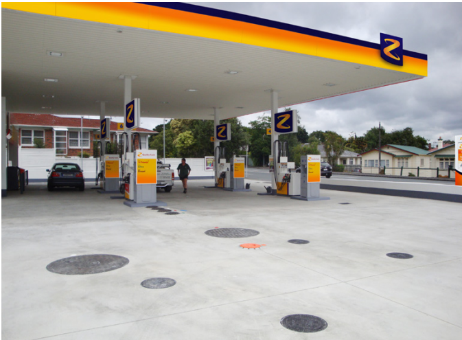
Recently upgraded site with Fibrelite's 1020mm covers (FL100) and 300mm covers (FL120)
