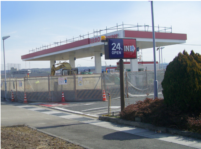
Site under construction
