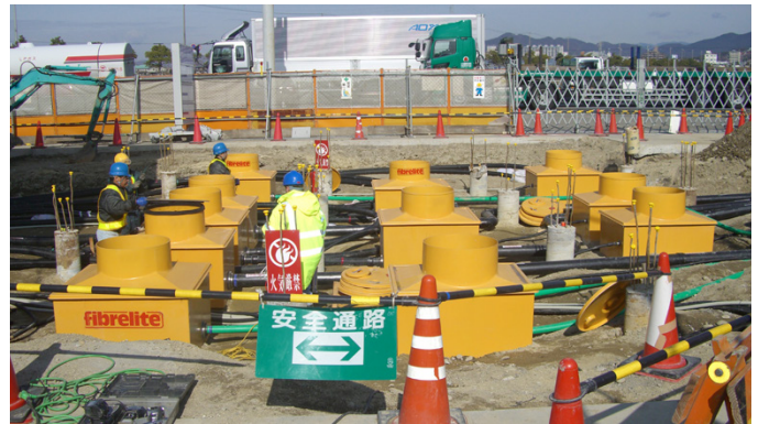
Vacuum tested tank sumps
