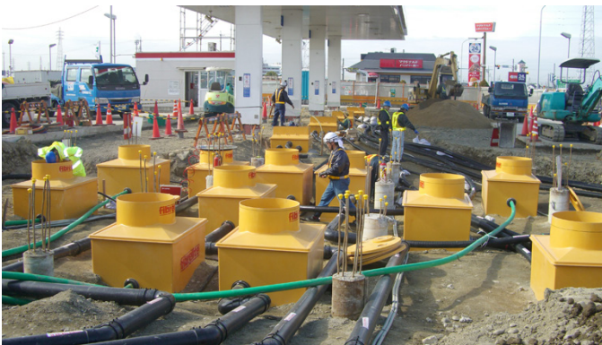
Fibrelite tank sumps and dispenser sumps being installed
