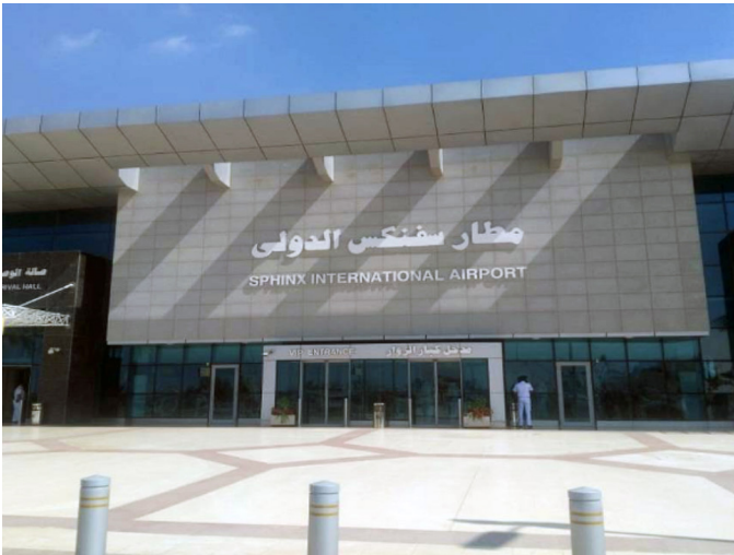
Sphinx Airport, Egypt install Fibrelite covers and chambers
