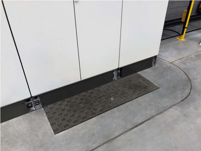
The Fibrelite covers that were installed could withstand loads up to 12.5 tonnes
