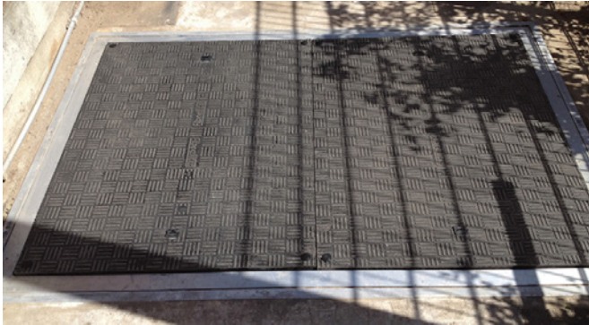
Sealed odour-tight covers installed
