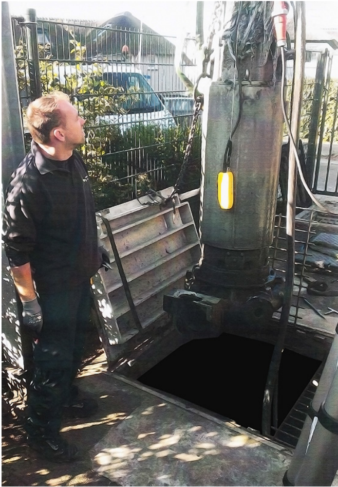
Heavy metal covers requiring 2 men and a crowbar to remove, emanating odours
