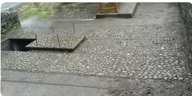
Cobbled covers requiring lifting equipment
