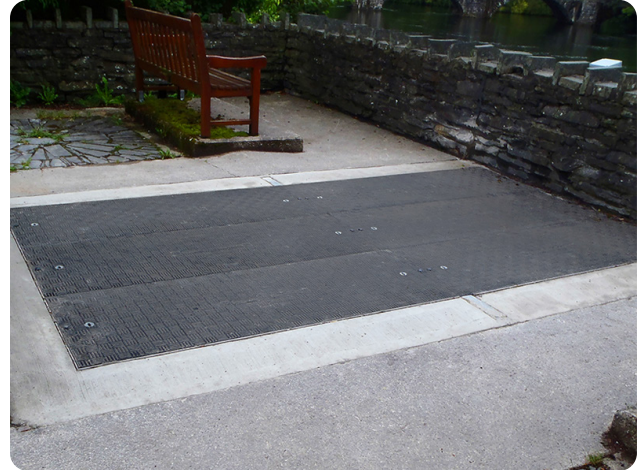
Lightweight Fibrelite trench covers now installed
